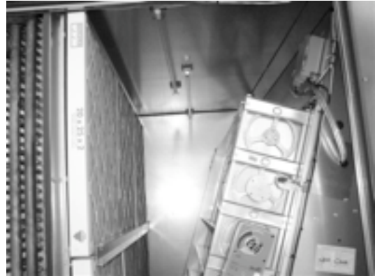
Return area of HVAC system before filter.
